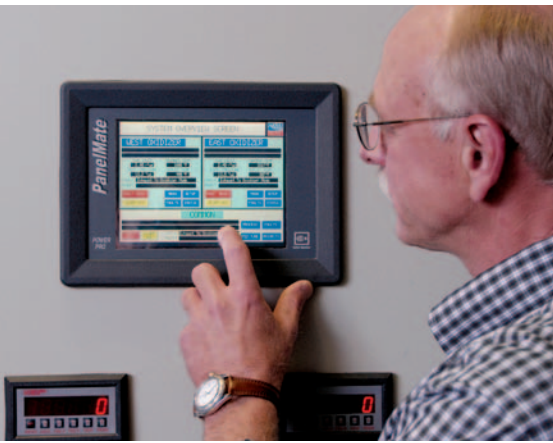
Programmable settings, fully-automated processes and minimal maintenance allow the thermal oxidizers to operate with minimum attention from Dean Veldboom and other Brown Printing staff.
