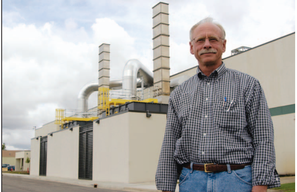
Dean Veldboom, facilities manager for Brown Printing, oversees the operation of two Regenerative Thermal Oxidizers (RTOs) for process emissions control. The impressive units are housed in a custom installation adjacent to the Waseca plant, shown in the background.
